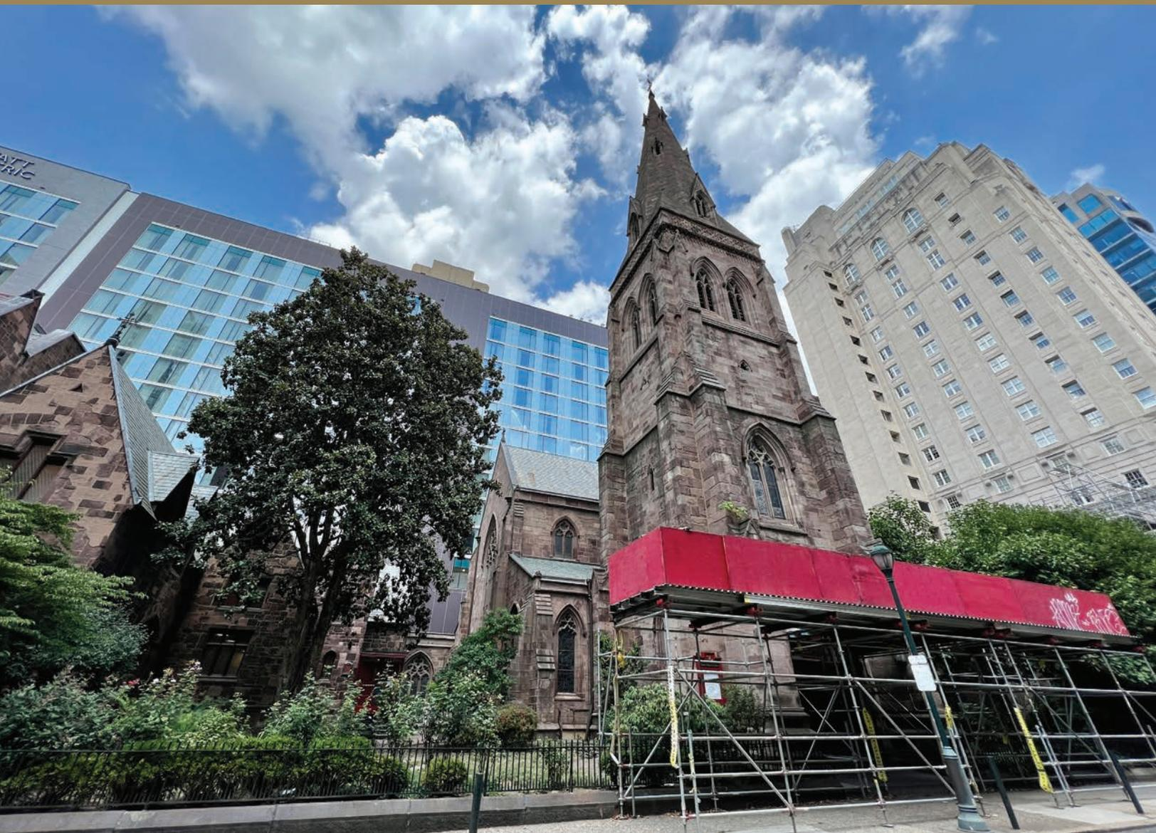
**B**rownstone is a kind of sandstone. It's sedimentary rock formed in layers, relatively soft, and prone to deteriorate in a number of ways as a result of its exposure to the elements over time.
